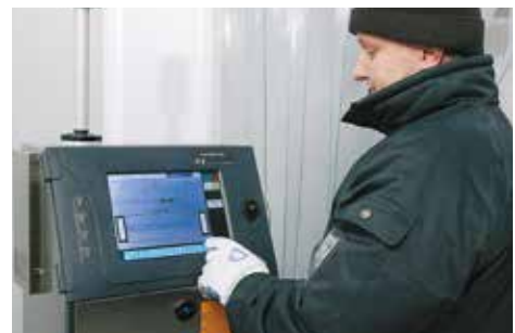
Installation i kylrum +4°C
